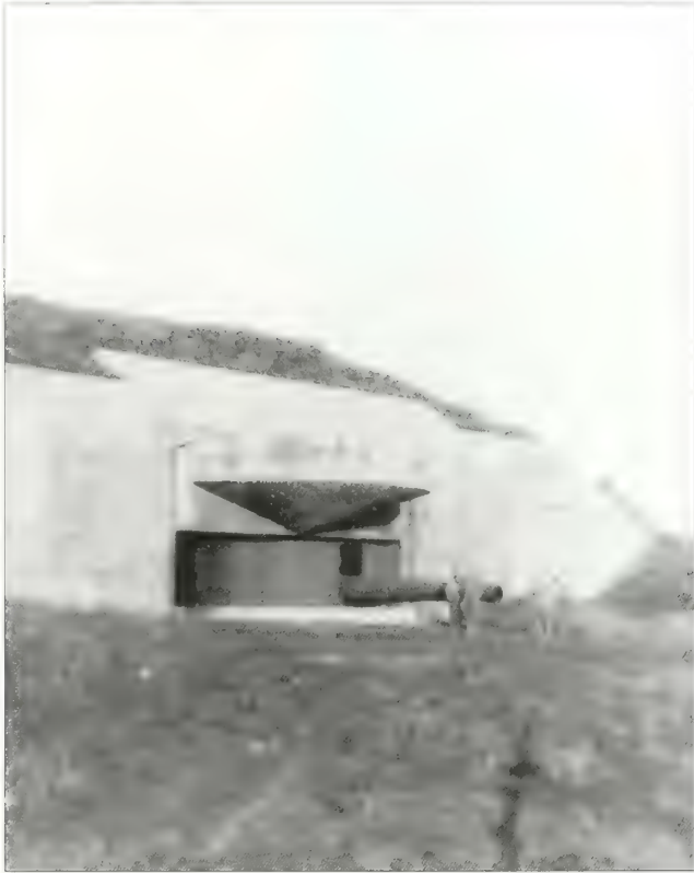
Figure 5.83. North gun emplacement, Battery Kingman, circa 1940s. This photograph shows the vegetation immediately around the gun emplacement and on the earthen casemate above was a low growing turf mixture ensuring the field of fire would not be obstructed (GATE 8085).
